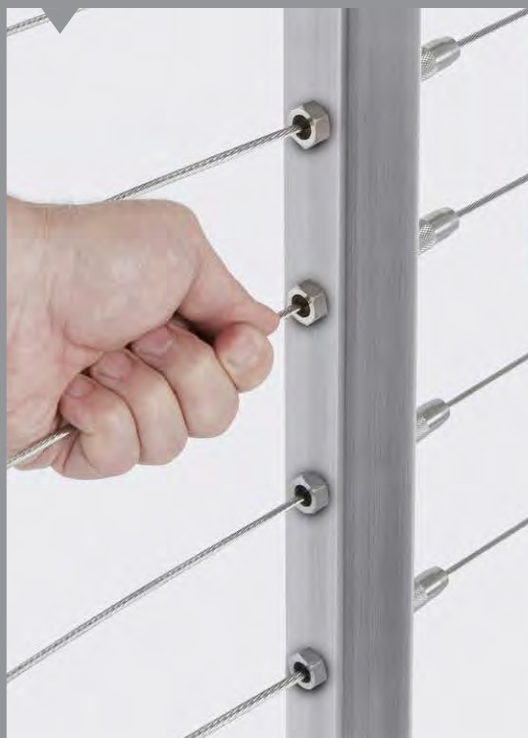
2. PULL CABLE THROUGH FITTING.
