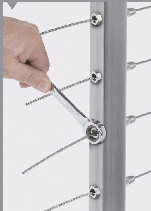
3. TENSION CABLE FROM EITHER END WITH A SINGLE TOOL.
