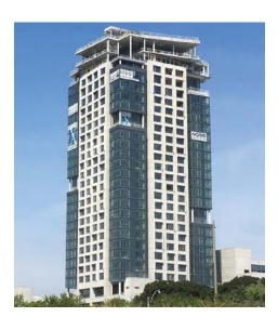
Che Hotel X guardrail configuration was tested successfully to wind loads of up to ±3.5 [KPa] (±73.1 psf).
