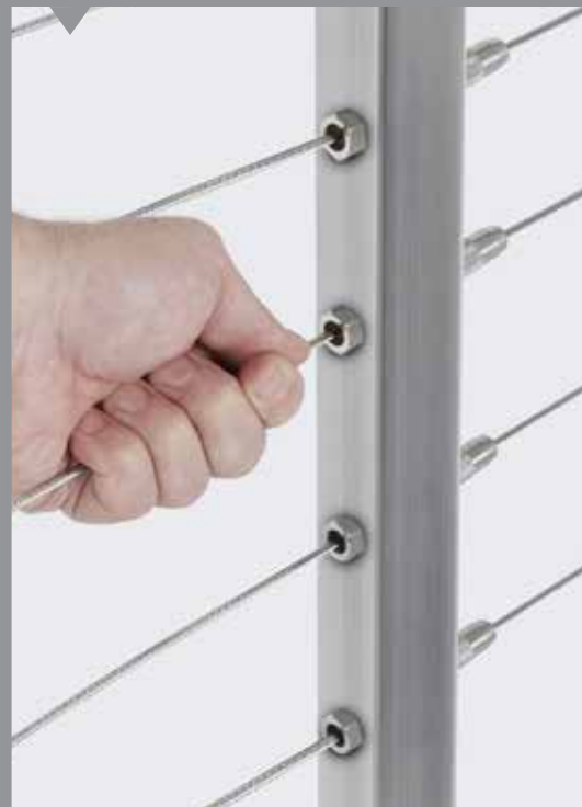
2. PULL CABLE THROUGH FITTING.
