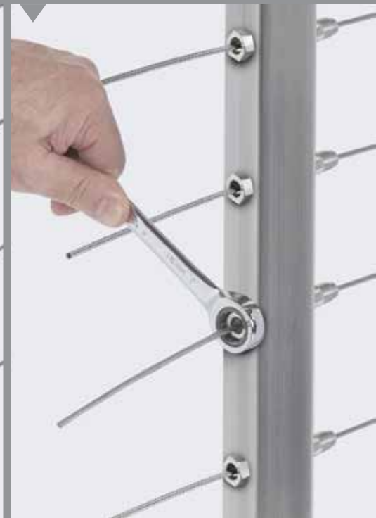
3. TENSION CABLE FROM EITHER END WITH A SINGLE TOOL.
