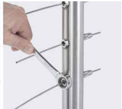
3. TENSION CABLE FROM EITHER END WITH A SINGLE TOOL.
